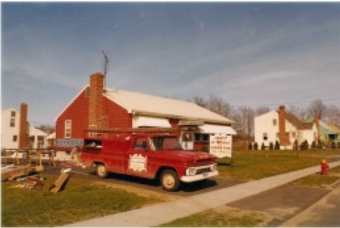
Early photo of a typical Peter L. Brown Company install
