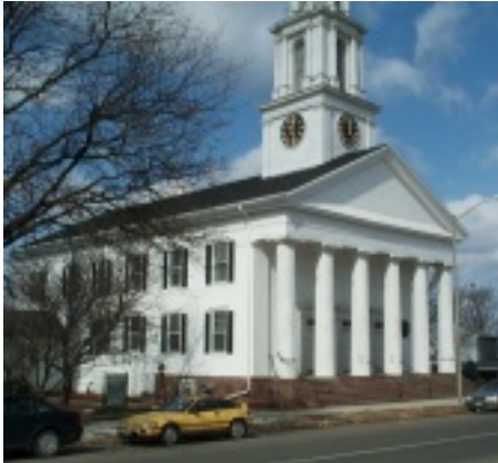
Churches, hospitals, historic renovations and other commercial endeavors are both challenging and rewarding
